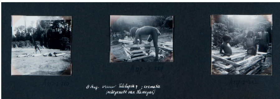
Figure 11. The preparation of the pyre for the cremation van Telelupta on Augustus 8, 1937 (from the photo album of Claudius H. de Goeje. Collectie National Museum van Wereldculturen. RV-A117-2).
