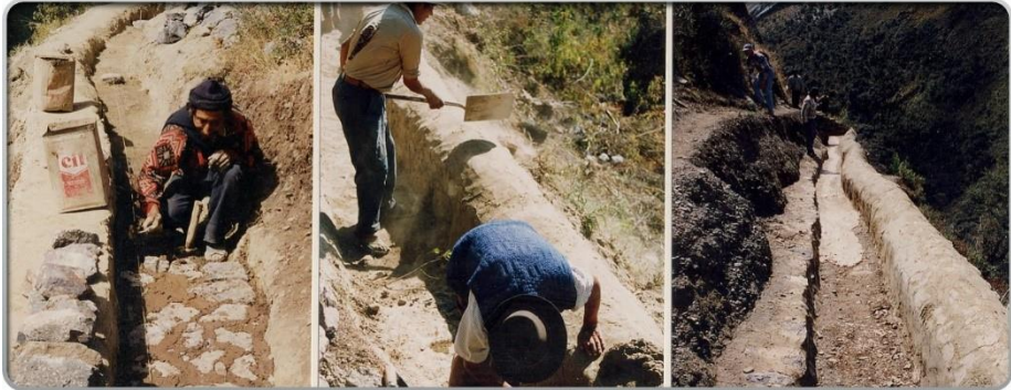
Photography 4. Triple photos of canal restoration work.
