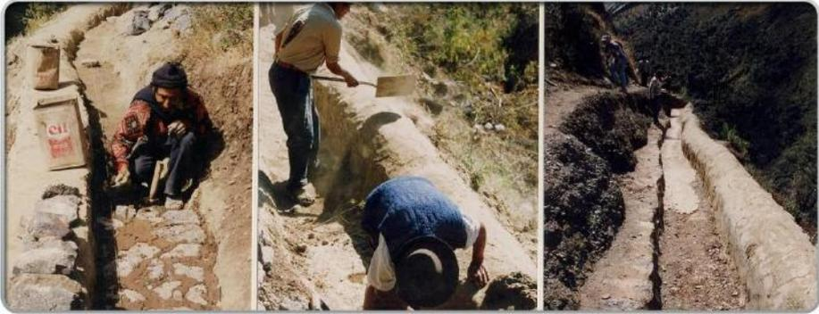
**Photography 4.** Triple photos of canal restoration work.
