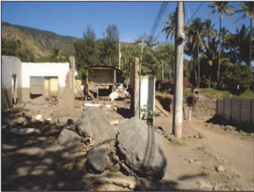
Figure 2. Damages created by lahars during the Hurricane Stan in the East flank of the Santa Ana Volcano in 2005.
